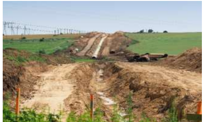
Figure 4. Underground Pipeline in Romania
