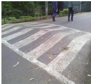
Figure 1. Concrete speed breaker
