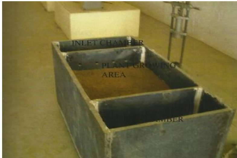
Figure 1. View of tank
